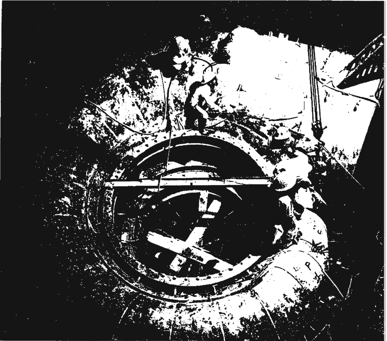
Installing one of the four giant turbines at the Hsianghungtien hydro-electric power station in Anhwei province. The turbines were made in Harbin, and the station was designed by provincial technicians.
